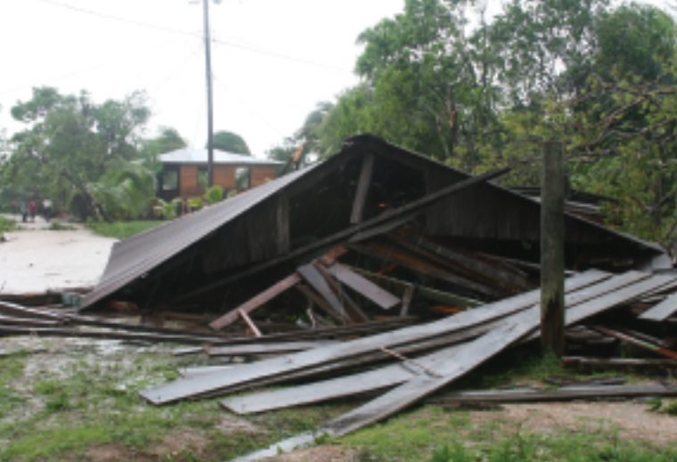
House destroyed by Hurricane Felix in Nicaragua in Sept. 2007. © CADPI
